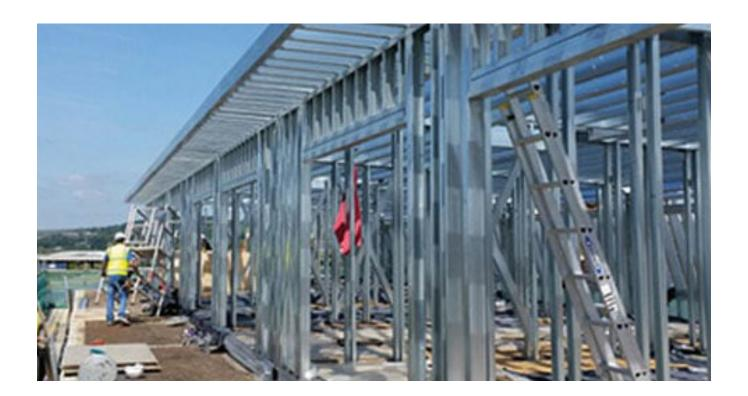
Located in a coastal area, this conversion from concrete frame building into exquisite riverside townhouses outlined strict specifications that required precision and expert delivery. A Frameclad steel frame system (SFS) was the ideal choice for the development.
