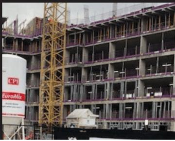
Frameclad's infill walling stud & track systems were installed to the primary structural frame of the buildings, providing support for the cladding system. Infill walls are considered to be non-loadbearing but resist wind loads applied to the facade and also support their own weight and that of the cladding. Light steel infill walls using C and U sections are increasingly being used for student accommodation above 18 metres.
